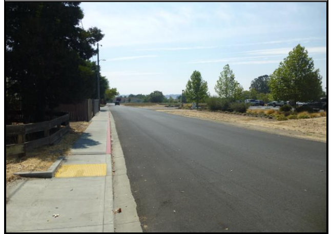
Looking south along 4 th Street.
